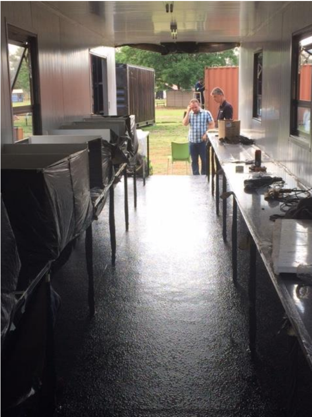
Installation of the cubicles:
